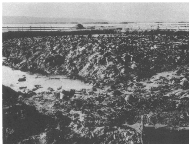
Figure 10. Artificial pond near Brest Merchant Harbor filled with oily debris which has been treated with quick lime
