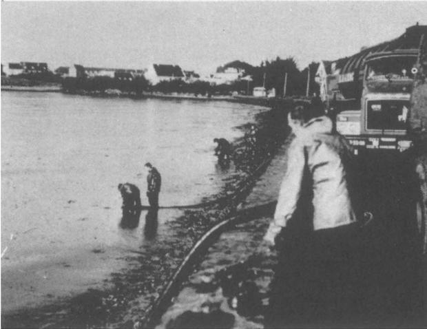
Figure 3. Pumping oil from the surface of the water using vacuum trucks near Portsall.
