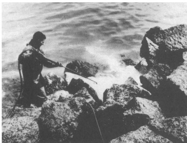
Figure 8. Cleaning of rocks using high pressure, hot water hosing technique
