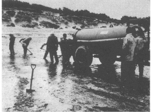
Figure 4. Pumping the oil trapped in a small beach pond by use of a "honey wagon's" vacuum pump
