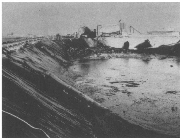
Figure 9. Artificial pond near Brest Merchant Harbor being filled with the more liquid portions of oily waste from the *Amoco Cadiz* spill
